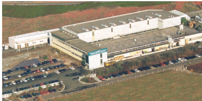
Headquarters of Walther Werke in Eisenberg, Germany
