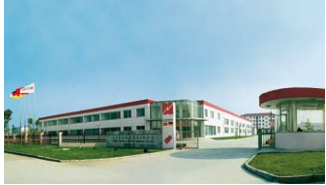
Nanjing works, productions facility to serve the Chinese market
